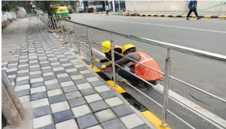
Phase-2 Police station road upgradation project completed in Peenya, Bengaluru
